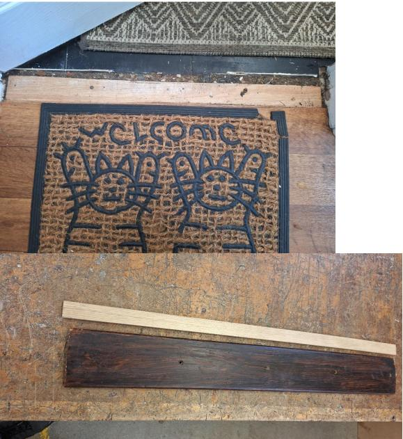
I had been putting off this job for a while, but it was something I had planned carefully. It's slightly curved and needed new pilot holes to sit the screw flush below the surface which is why I added 1mm clearance to the diameter.
